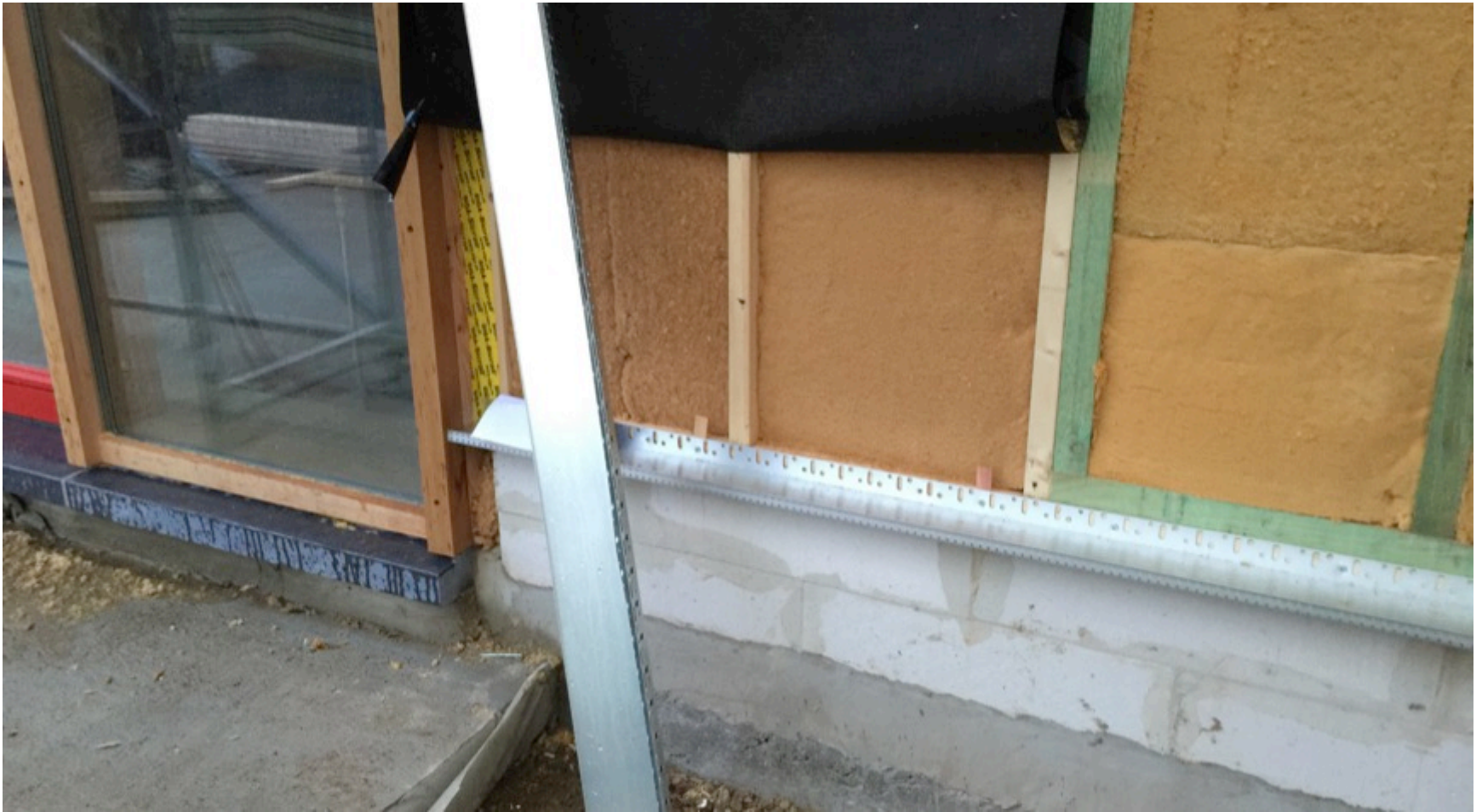
External insulation with wood fiber
